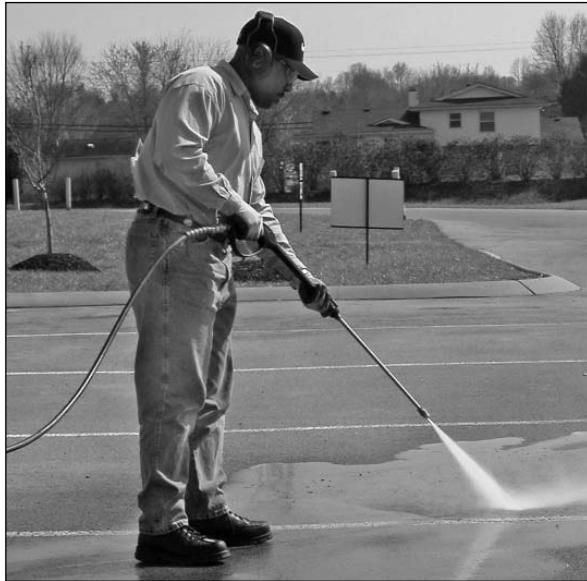
Figure 15 - Optimum angle to cleaning surface
